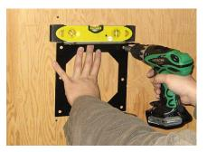
Mount the WSB at the desired location using the four (4) 1/4" x 1 1/2" bolts supplied. If mounting on brick, stone or stucco, masonry anchors or other mounting hardware may be needed. Legendary Lighting does not supply masonry anchors.
