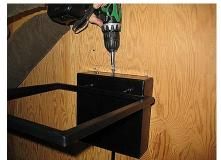
After connecting to gas and/or electricity, rotate the lantern bracket into final position and install one bolt at top center and one bolt at bottom right. If a top curl is
